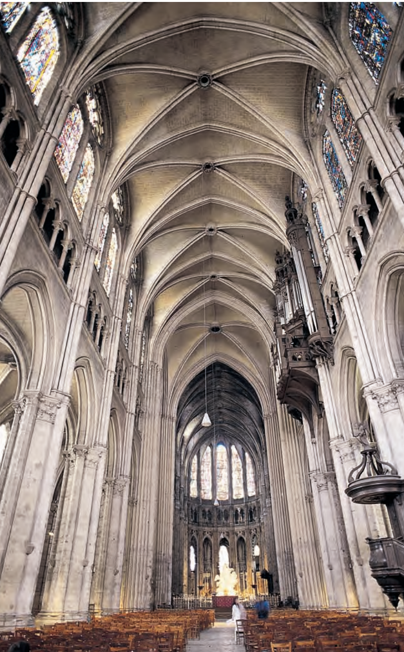
13.18 Nave, Chartres Cathedral, looking east. The three stories of Gothic elevation rise on either side of the nave. The lowest story, or nave arcade, is defined by a series of large arches on heavy piers. These separate the nave from the side aisles (see fig. 13.12). The second story, or triforium , is a narrow passageway above the side aisle. At the top is the clerestory, whose windows are the main source of light in the nave.
