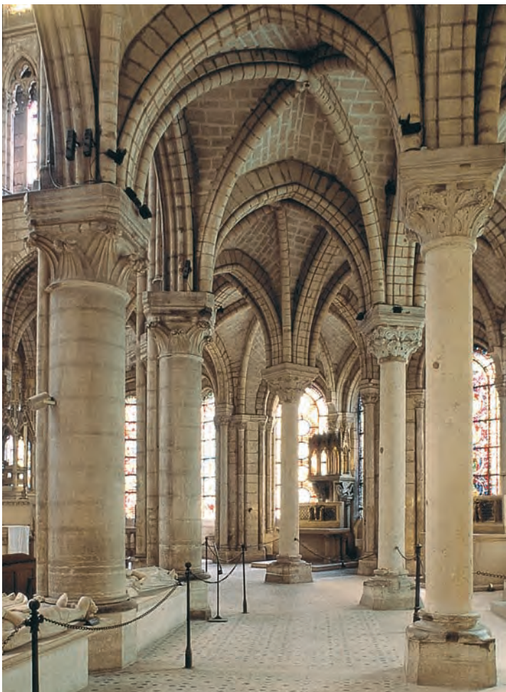
13.2 Interior of Saint-Denis. Each chapel bay has a pair of large stained-glass windows, delicate columns, and rib vaults. The ambulatory and chapels have merged to form a series of spaces illuminated by large windows supported by a masonry frame. Suger described the new effect as “a circular string of chapels, by virtue of which the whole [sanctuary] would shine with the miraculous and uninterrupted light of the most luminous windows.”
