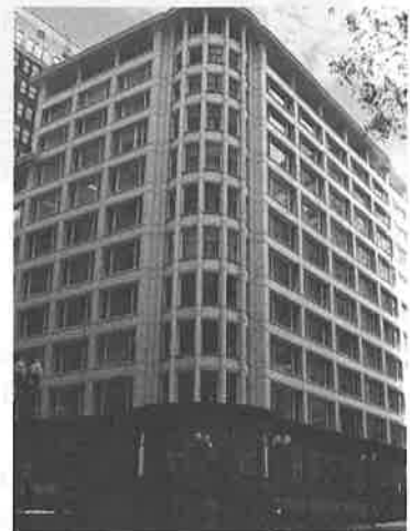
Figure 21.14a: Louis Sullivan, Carson Pirie Scott, 1899–1904, iron, steel, glass, and terra-cotta, Chicago
