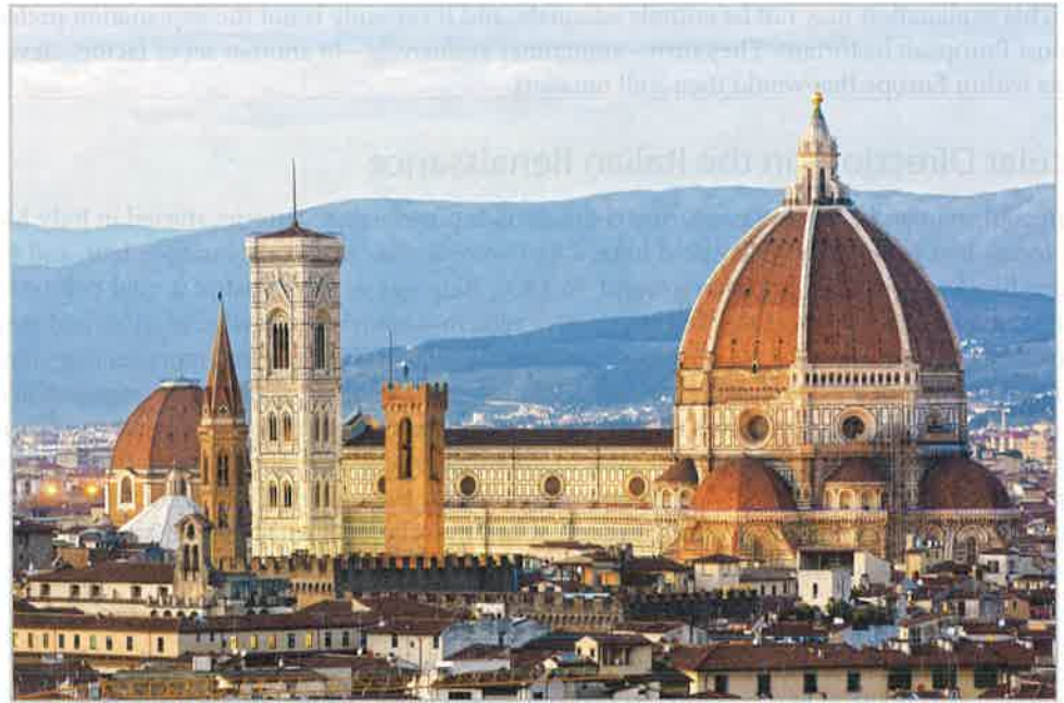
FIGURE 16.3 Although the nave of Florence Cathedral was completed in the fourteenth century, it was not until the fifteenth century that architect Filippo Brunelleschi was able to solve the engineering challenge presented by the plan for the massive dome. In order to eliminate the need for temporary wooden scaffolding during construction, Brunelleschi used a skeleton of eight large ribs alternated with eight pairs of thinner ribs, all tied together by nine sets of horizontal ties, all of which would be able to support the workers as the dome was raised.
