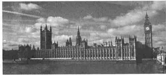
Figure 20.1a: Charles Barry and Augustus Pugin, Palace of Westminster (The Houses of Parliament), 1840–1870, limestone, masonry, and glass, London
