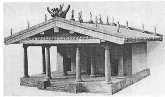
Reconstruction of an Etruscan Temple of the 6th century according to Vitruvius
